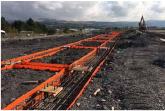
Foundations under construction.
