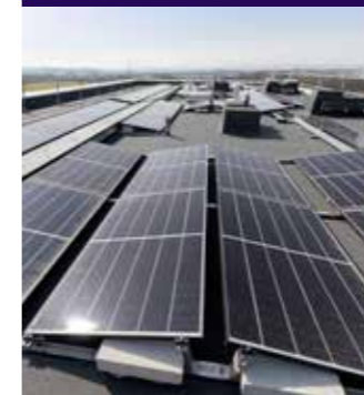
Integration and Collaborative Working Award George Parker Bidder Building, Exeter Science Park
