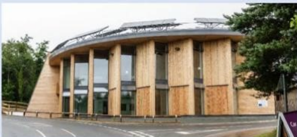
Green Build Hub, Eden Project
