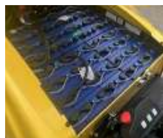
Electric forklift truck battery pack. Bradfords added 27 of these to its fleet in 2023.
